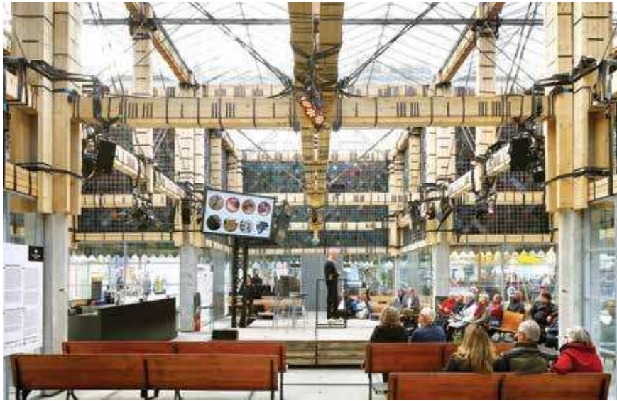
The glass roof was made using a system that is commonly employed in the greenhouse industry. Courtesy of Filip Dujardin, v2com
